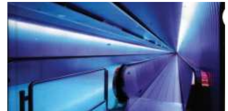
Frankfurt Airport Tunnel 1997-2007
